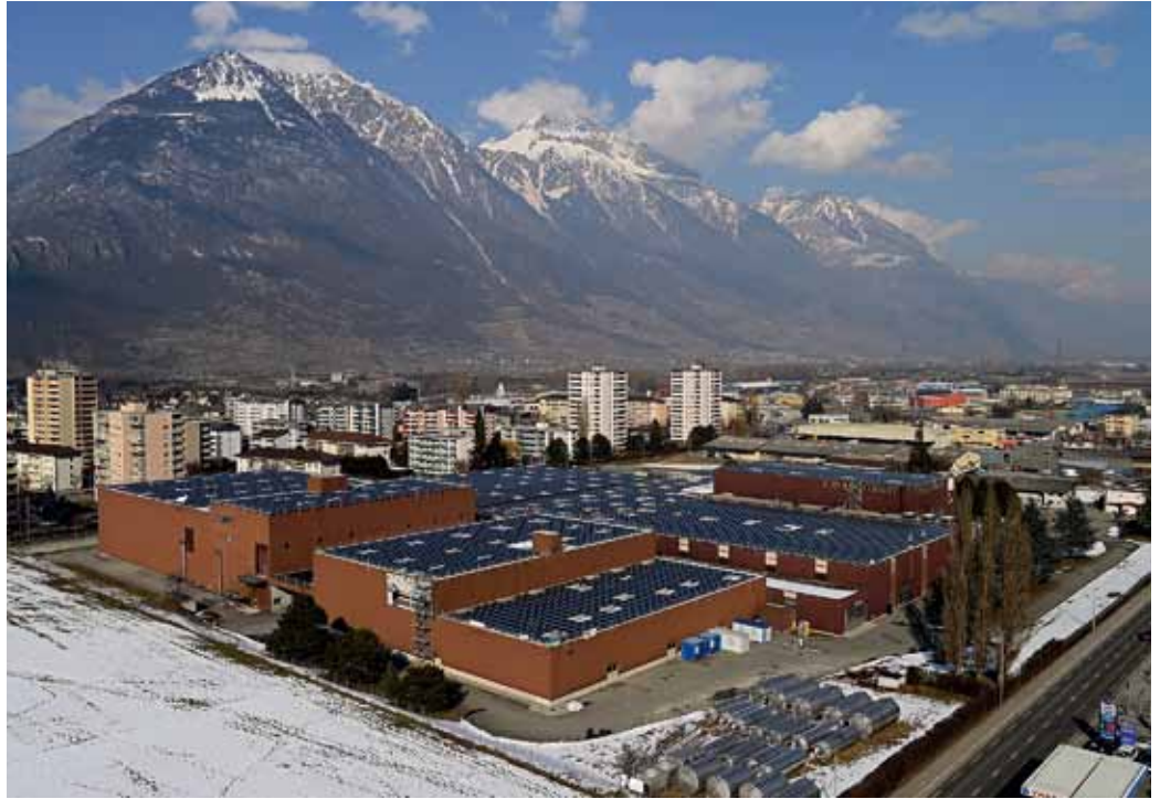
Helle Freude: Fotovoltaik-Anlage in Martigny.
