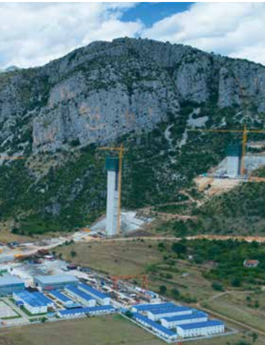
Autobahnbrücke in Montenegro.
