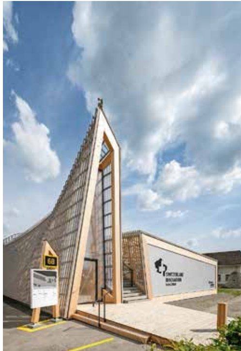
Blamage: Innovationspark in Dübendorf.
